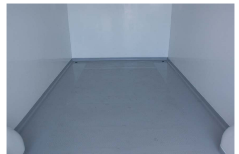
Interior Showing 75mm edging on floor and one piece panel construction
